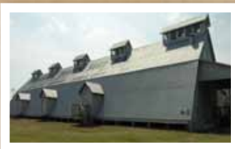
January 7, 2011: Seed Warehouse No. 5 at the southwest corner of US 165 and AR 161 in Scott. Constructed in 1948 by prominent cotton farmer Robert L. Dortch, Seed Warehouse No.
