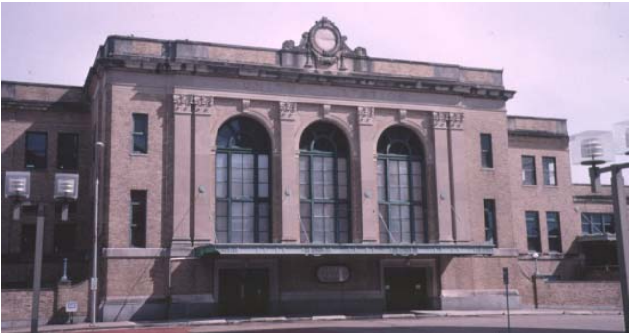
Texarkana Union Station, Texarkana, Miller County. AHPP Photo.
