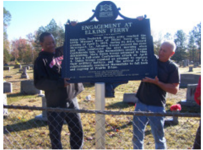
Installing the Elkins' Ferry/Cornelius Farm marker
