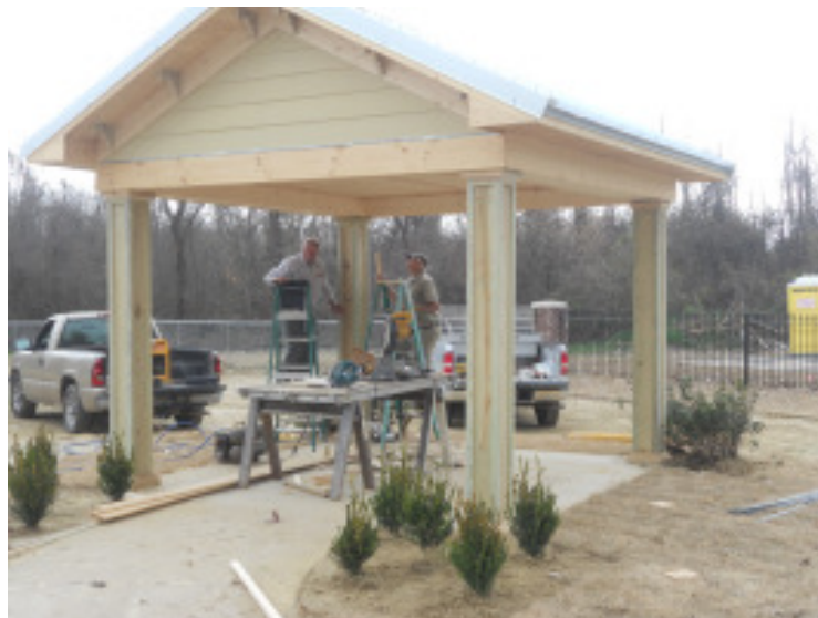
Workers construct a pavilion at Helena-West Helena's "Freedom Park" display
