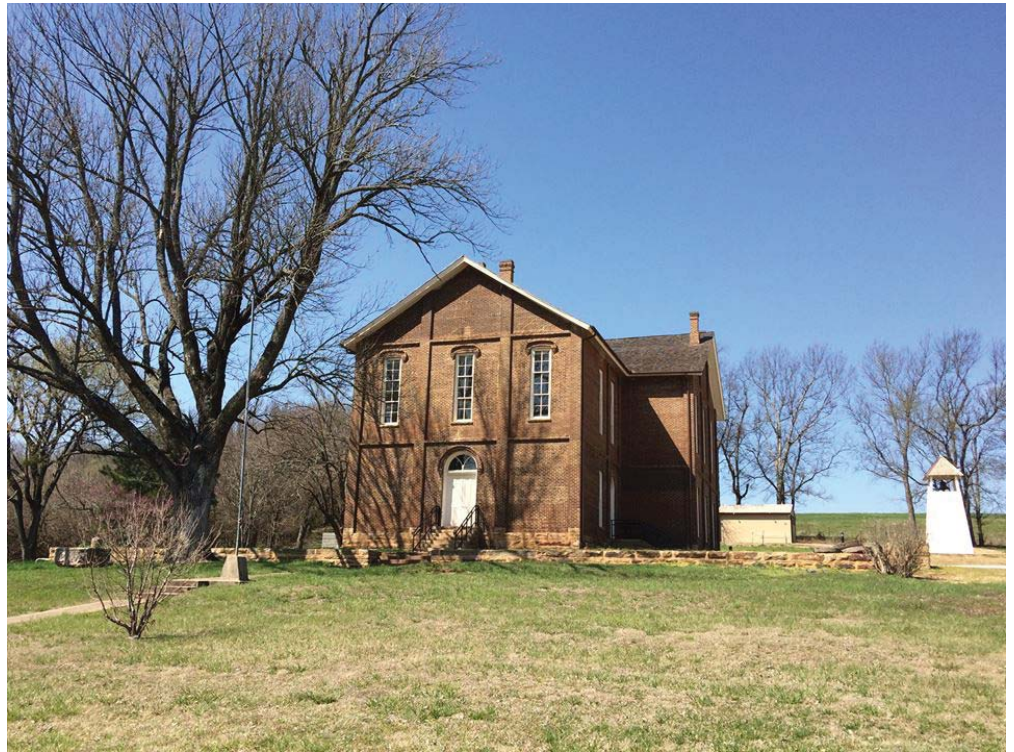
Cane Hill College building following its restoration
