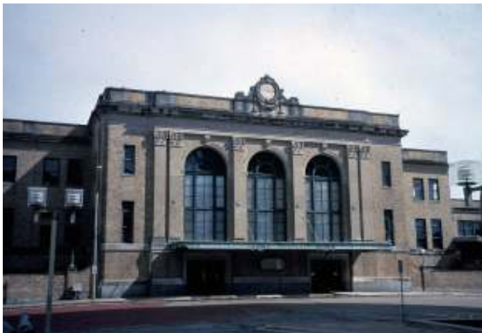
Texarkana Union Station and train platform
